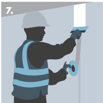
7. Taping and jointing for a seamless finish.
