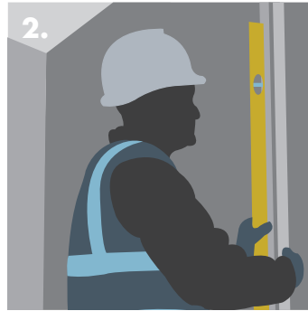
2. Fixing Knauf 'C' Stud to form the partition frame abutment.
