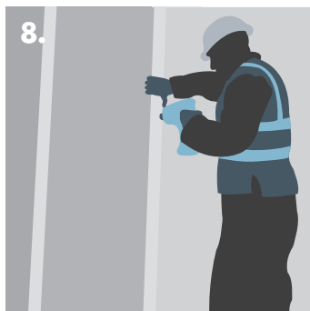
8. Fixing Knauf Plasterboard to the completed framework.
